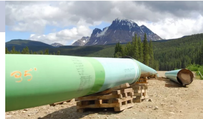
Pipeline under construction in Alberta, Canada | rblood via Flickr, CC BY-NC-ND 4.0
